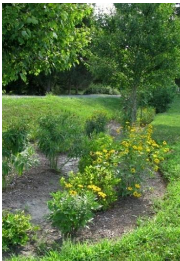
Environmental Site Design techniques, such as this rain garden, are required by the new stormwater management regulations.
