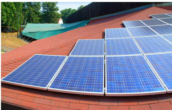
Solar panel demonstration projects are located on a number of Howard County facilities. They save energy and promote sustainability.
